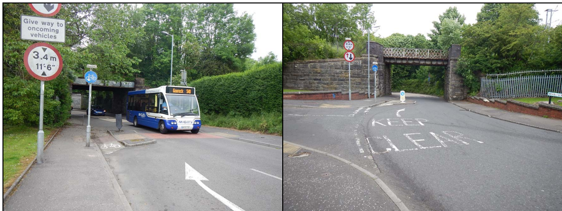
Figure 3.11 : Build Outs on Bridgend Road at the North and South Bridge AM Period
